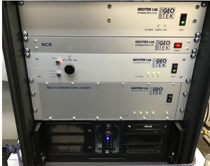
Figure 3.1: MSCL-S Schrack cabinet containing PC and electronics racks
